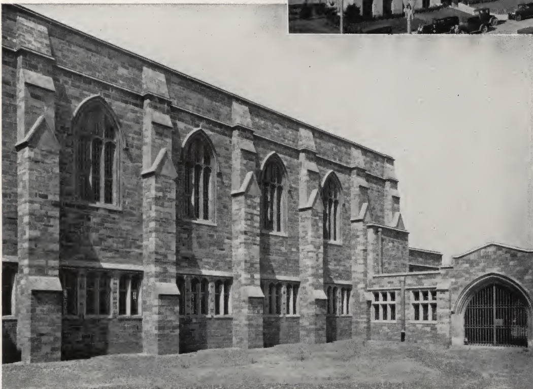
Above —Harborview Hospital at Seattle, Washington, owes its strength and safety to a reinforced concrete frame and 175,000 units of concrete masonry backup. Thomas, Grainger and Thomas, architects. Western Construction Co., contractor.
